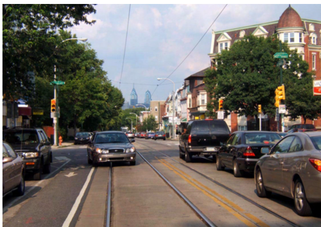
Baltimore Avenue, a principal arterial in Philadelphia, was striped with 10 ft. travel lanes to enable the installation of bike lanes. The effective curb radius of this intersection is significantly increased by the presence of the bike lane – as well as the parking lane – enabling motorists from the side street to easily turn right into the 10 ft. lane.
