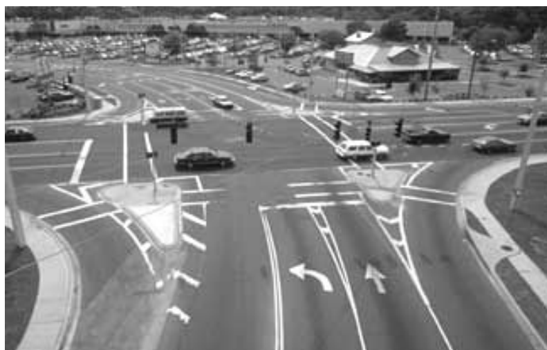
Figure 7.10. The design of channelization islands for slip lanes at intersections can be made more pedestrian friendly by changing entry angles and corner radii. Sources: Walkinginfo.org (graphic); Dan Burden (photo).
